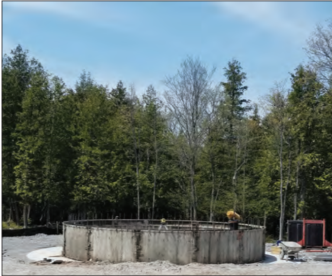
Construction of the Elevated Storage Reservoir Base.
