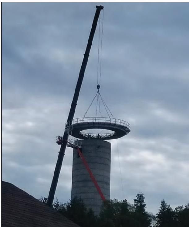
Lowering of the Elevated Storage Reservoir Pedestal.
